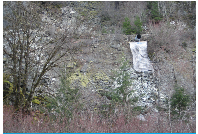
Custom CC drape for water overflow
