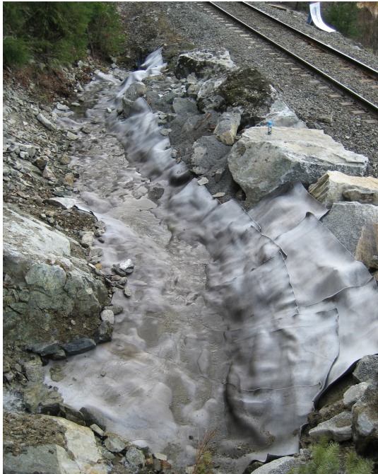
CC laid to direct water to culvert
