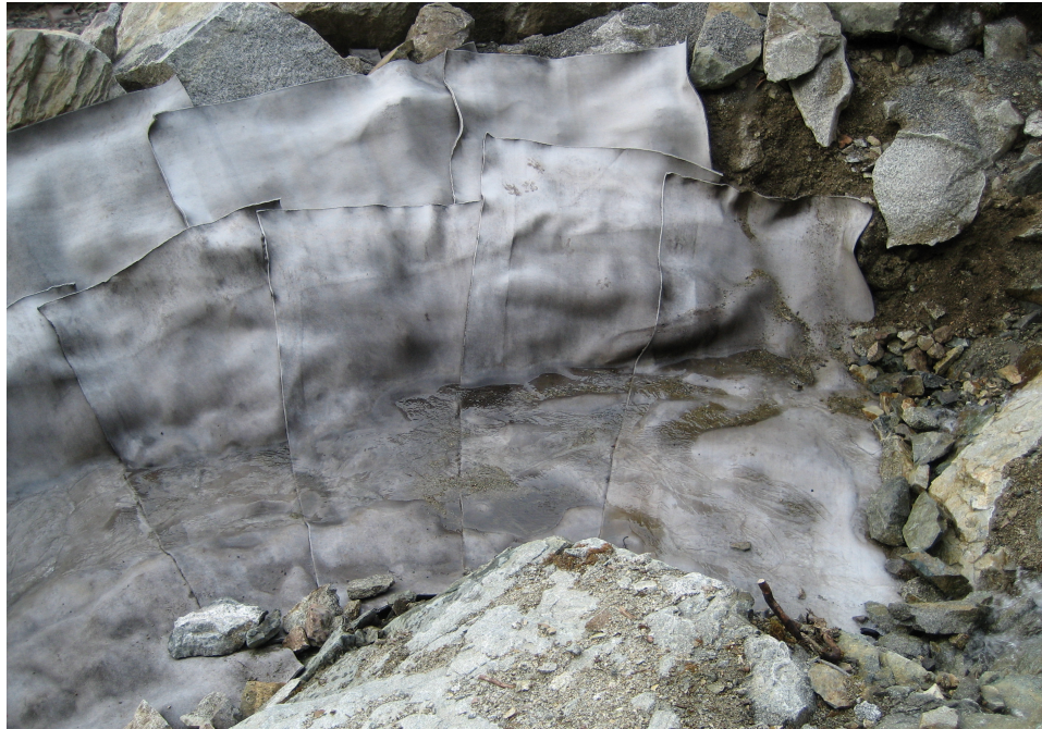
Extra layers of CC to protect track
