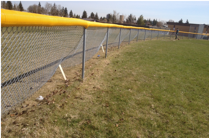
Site preparation before installation
