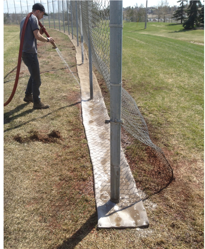
Hydration of installed CC
