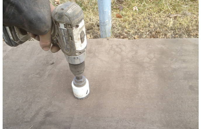
Drilling holes for placing CC around fence posts
