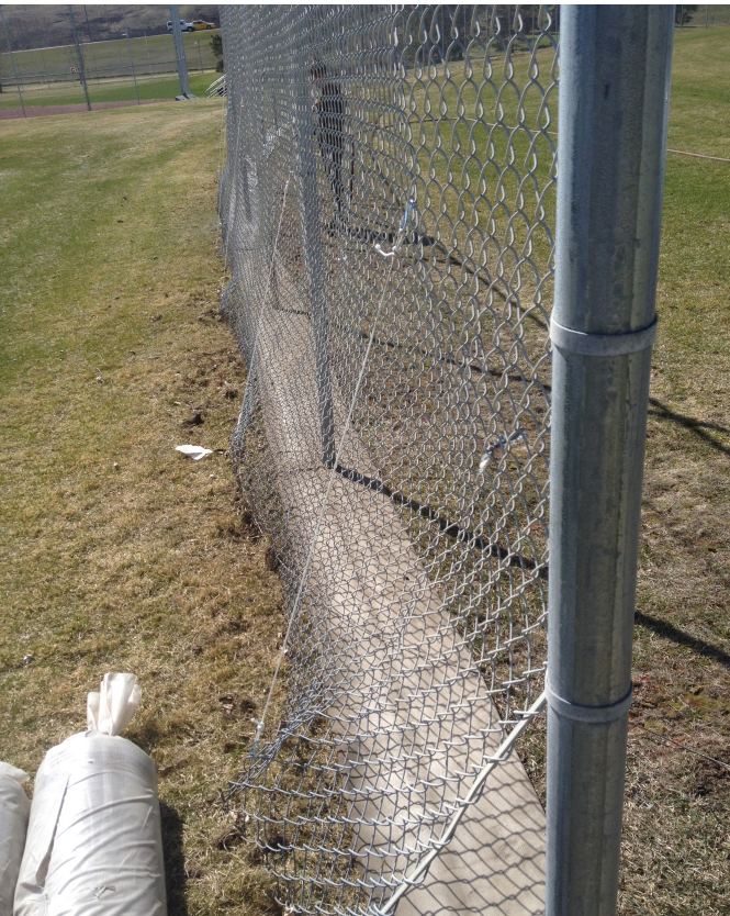
Fencing moved out of the way for installation
