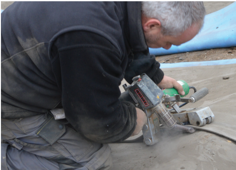
Thermal welding on the CCH joints
