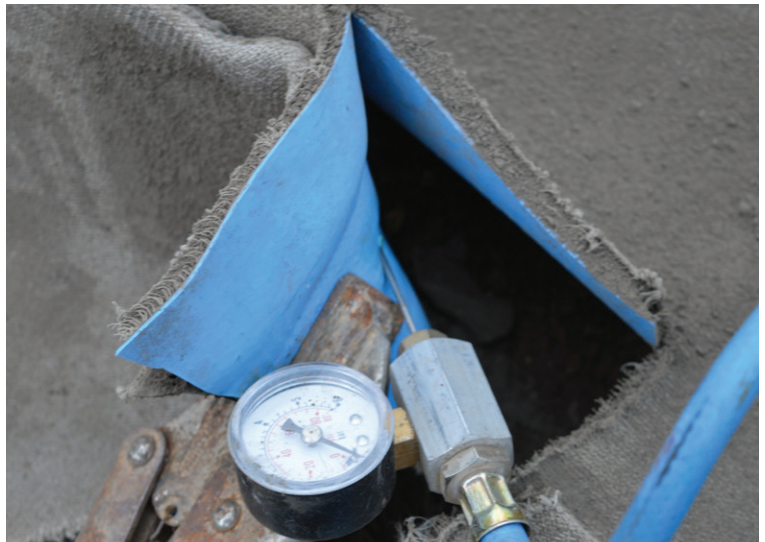
Pressure testing of the welded joints
