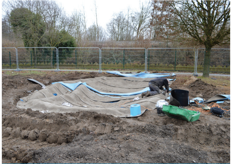
The CCH was laid transversely across the ponds
