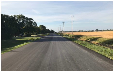
Spartan Road Grid™ 10 completed overlay on Peony Bay North Stt.
