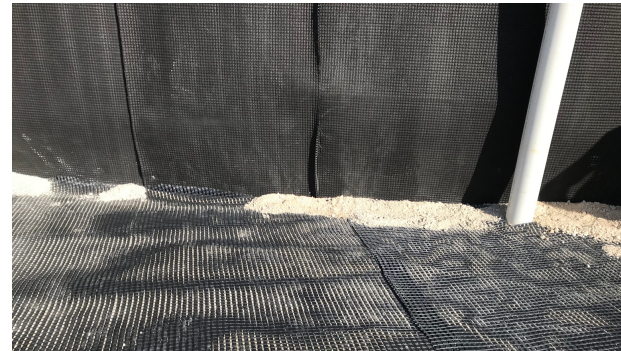
Deployment of roll layout of Pyramid Grid™
