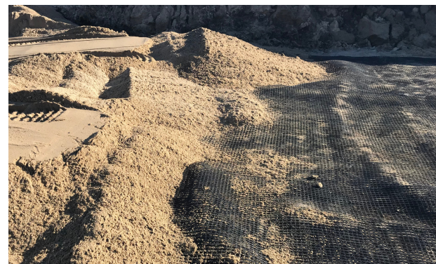
First layer of Pyramid Grid™ with granular
