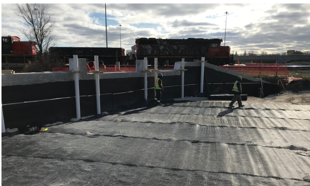
First layer of Pyramid Grid™
