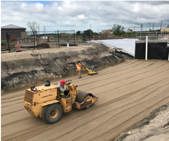
Pyramid Grid™ installation with granular compaction.
